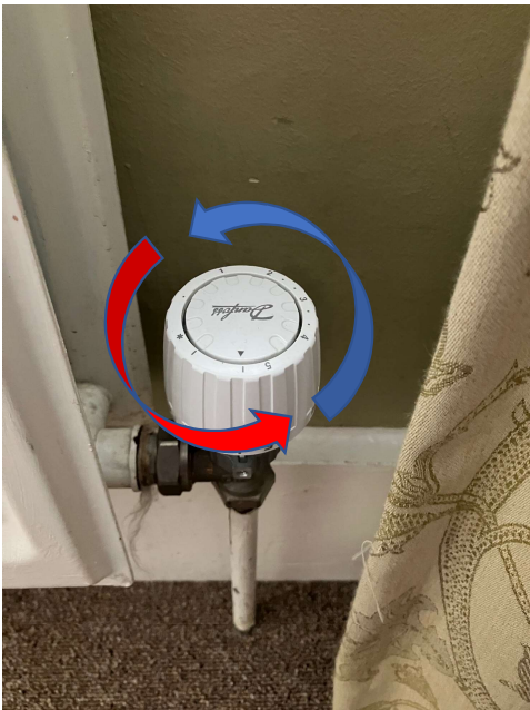
Radiator valve – use to adjust heat
